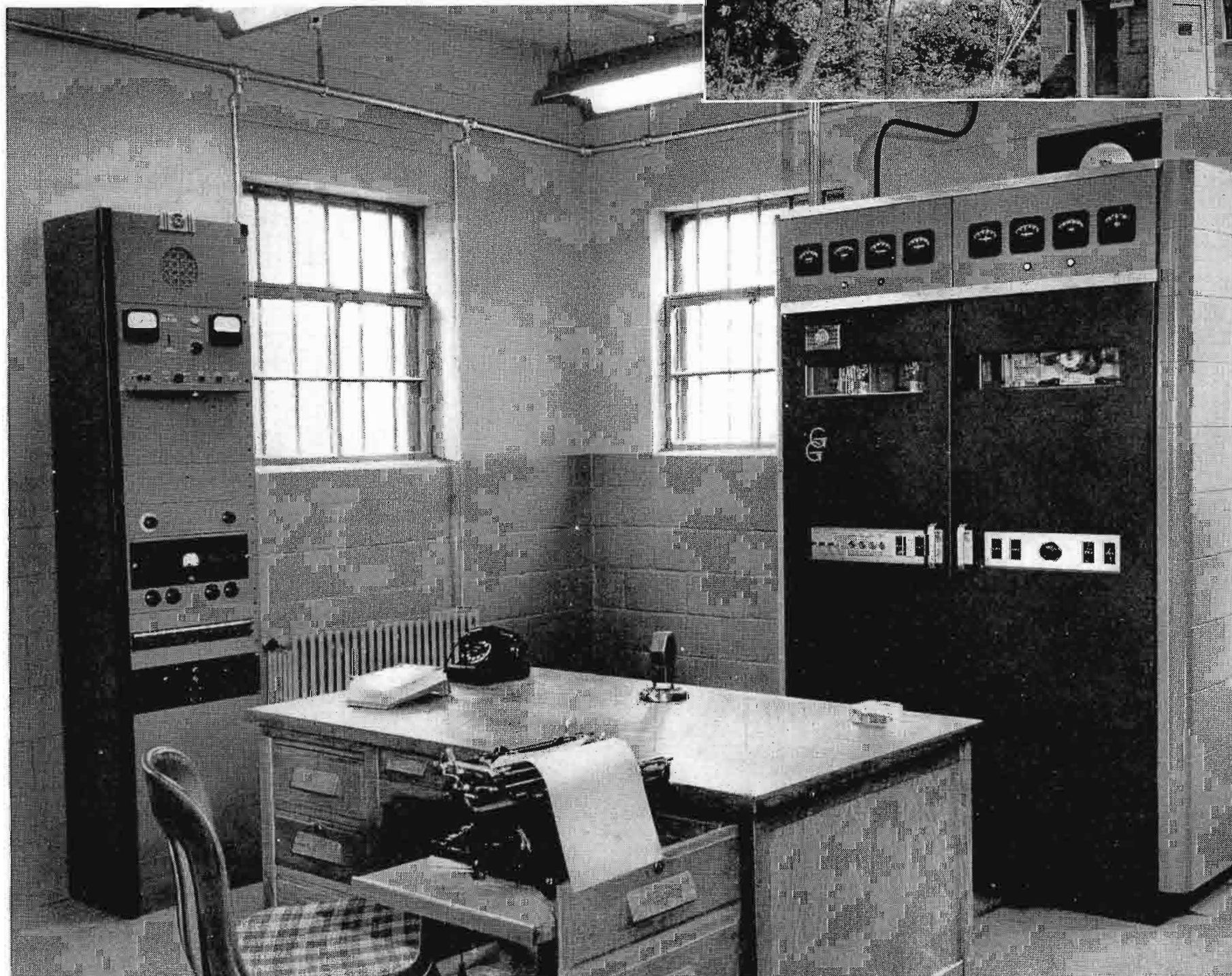
FIG. 3 (below). WRAK-FM's RCA transmitter and associated line and monitoring equipment are arranged primarily for convenience and accessibility.
